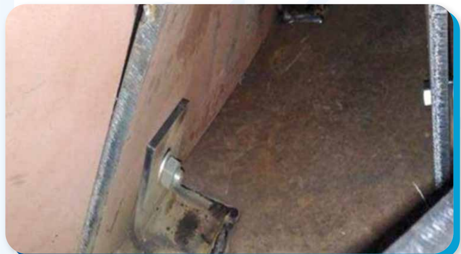
Figure 20 . Bolted-on components installed in a drum dryer.
